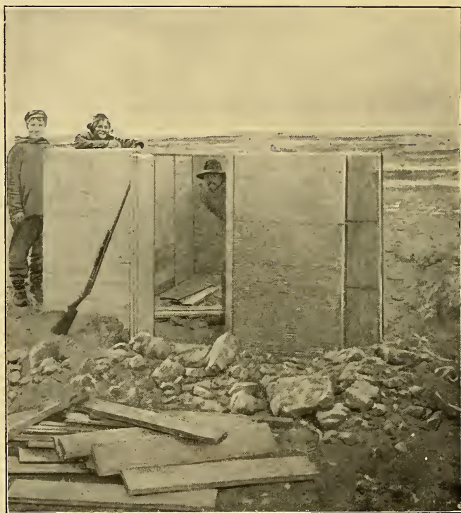
BUILDING THE MAGNETIC VARIATION HOUSE. GJÖAHAVN, 1903.
